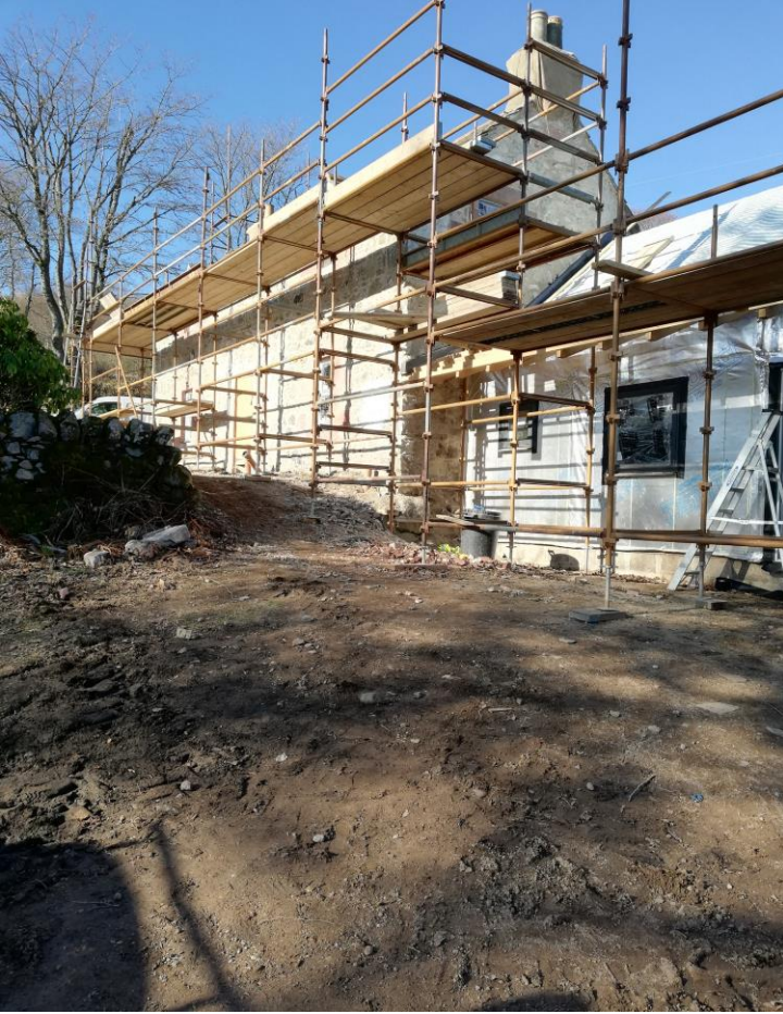
Unpainted rubble stone facades
